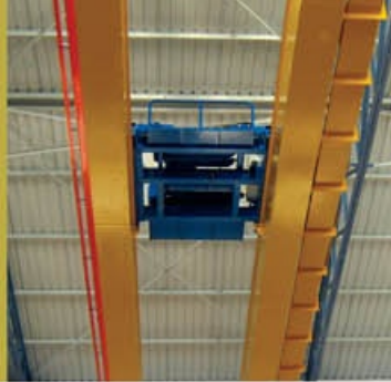
Double Girder Trolley Hoist
